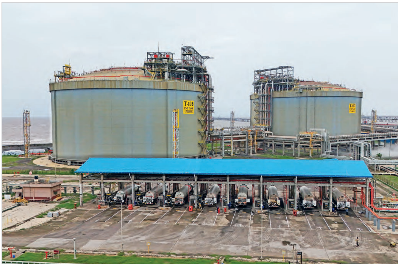
Truck Loading Facility (TLF) at Dahej LNG Terminal
