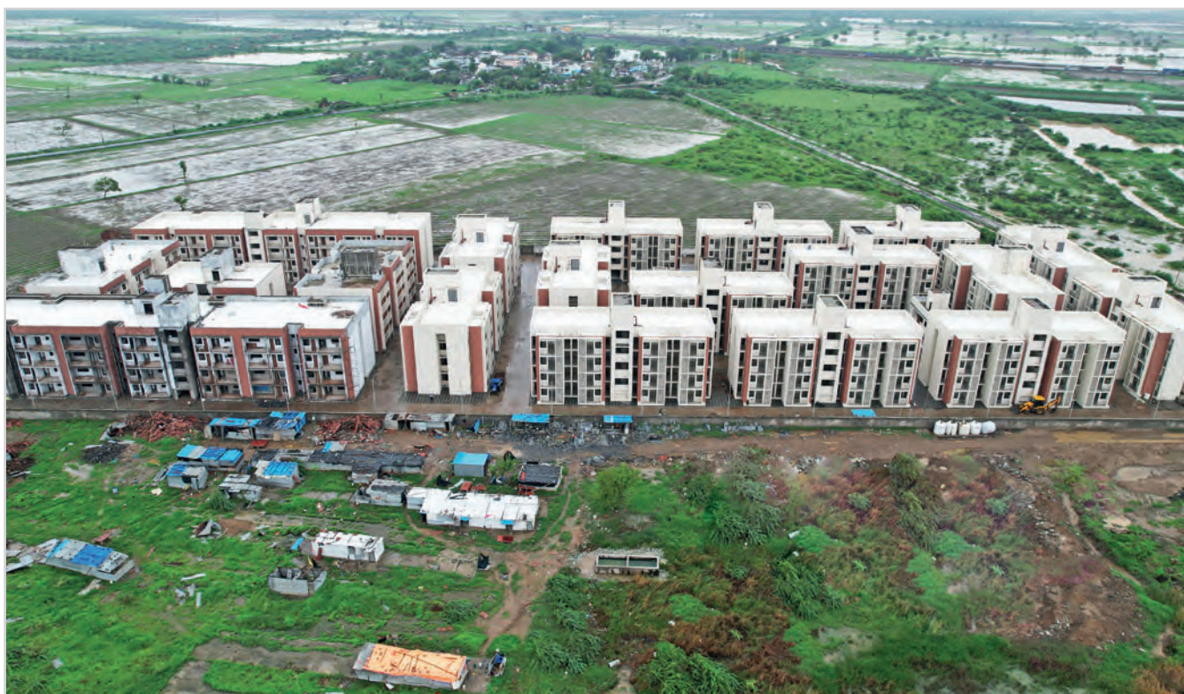
ARHC constructed by PLL at Eksal Village, Bharuch (Gujarat)
