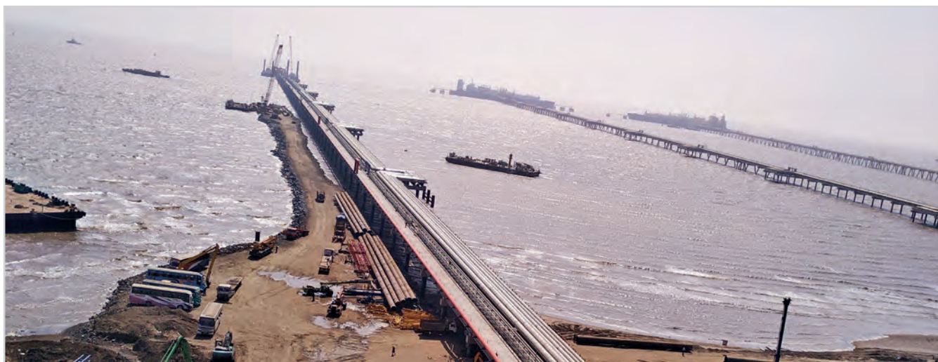
Construction of Third Jetty at Dahej LNG Terminal – A Strategic Addition to India's LNG Ecosystem
